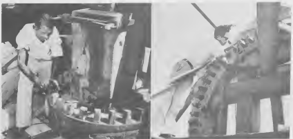
STUDY WOOD gears, left, probably part of the original mechanism, are re-installed by a workman. Evidencia of the hand work that went into beams and gears can be seen at right. APARATONAN DI palo pia, banda robes, probablemente parti di e mecanismo original, ta worde re-instala door di e trahador. Evidencia di e obra di man cu a bai den e molina por worde mira na banda drechi.
